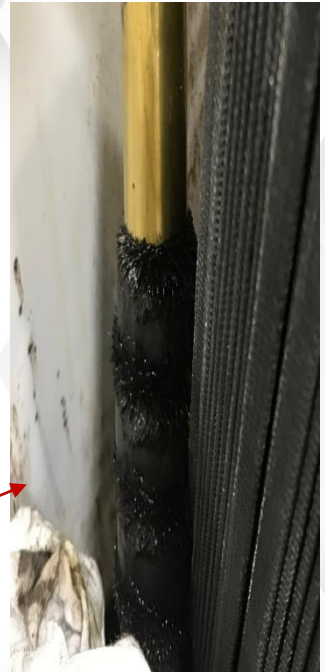
Magnetic Filter Rod
