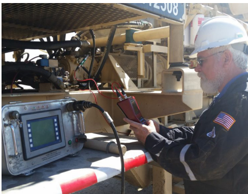
Onsite Troubleshooting & Repair
