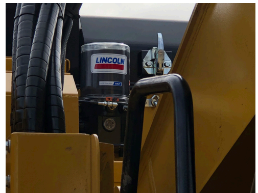
Lubrication System Installation & Repair
